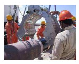
The pipes, used to carry out pipelines, should pass through specific processing phases such as welding and coating with shrink sleeves or epoxy powder fusion. All these operations must be carried out at higher than ambient temperatures, therefore the pipeline must be heated.
